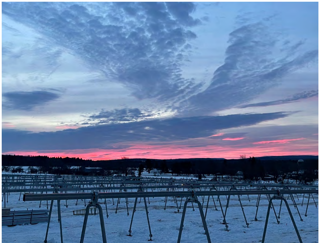
Figure 13: North Bangor site installed with TerraTrak.
