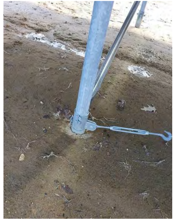
Figure 11: Real-life example of ground screw performance in a site pre and post frost heave
