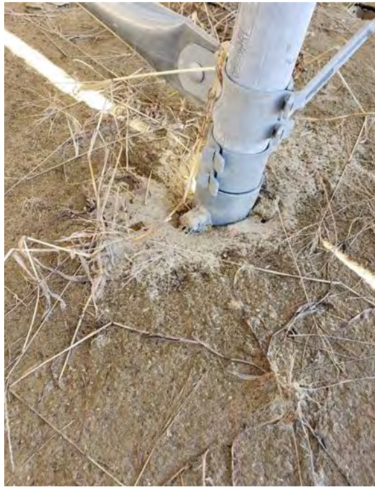
Figure 11: Real-life example of ground screw performance in a site pre and post frost heave
